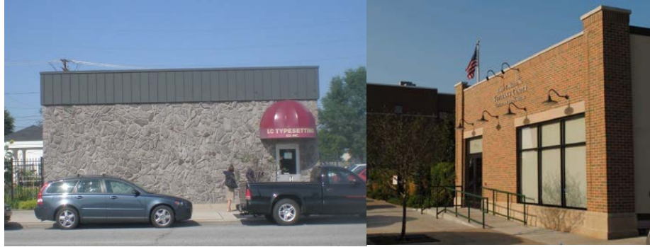
Original typesetting building at 747 S. Michigan Street and façade of new Veterans' Center completed in 2011 (Buccellato Design, LLC). Images: Author
