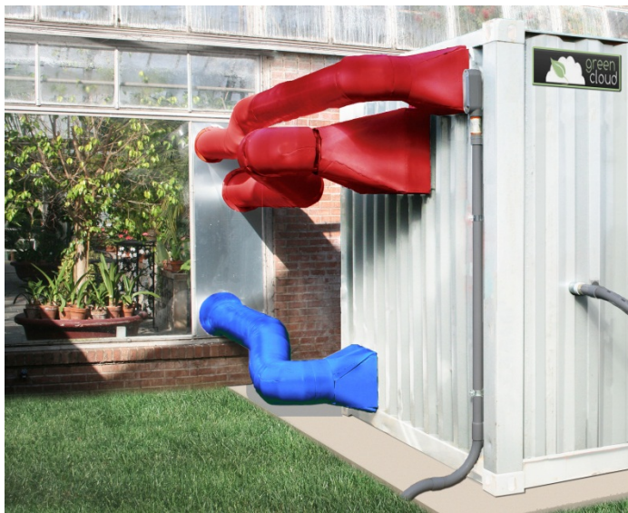
Image 4: Visitors to the Conservatory will be able to see the mechanics of the Green Cloud concept from inside the Conservatory and out. This image shows the ductwork that connects the Green Cloud to the Conservatory painted red and blue to indicate how heat is delivered from the servers to the building. Image credit: S. Santeramo.
